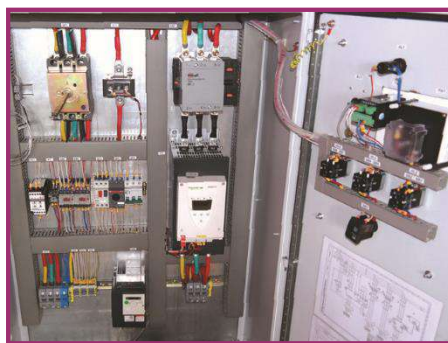
Control cabinet with frequency changer
